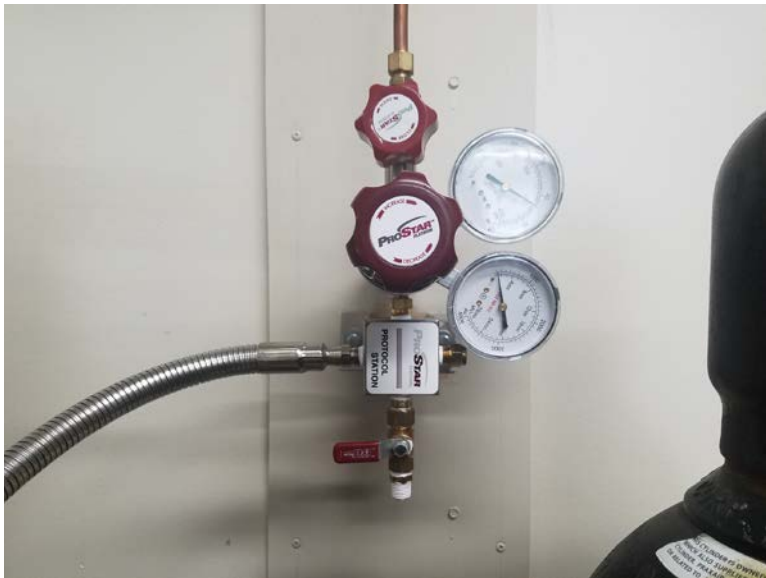
Close main valve leading to glove box
