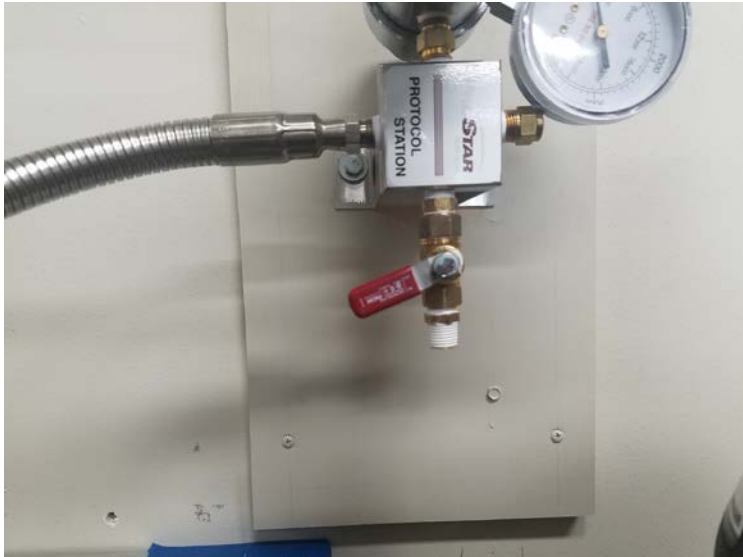
Vent gas line using bottom valve (15 sec)
