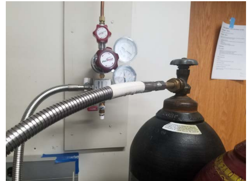
Connect to nitrogen tank and open tank valve
